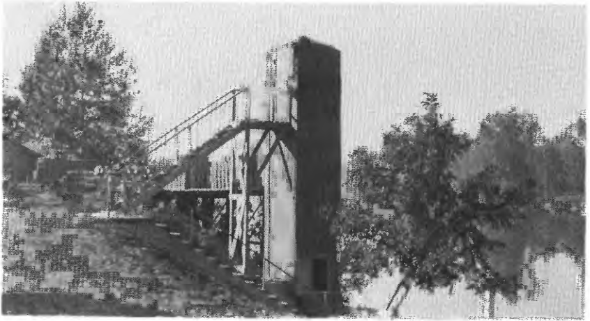
B, WILLAMETTE RIVER AT ALBANY, OREG. FIGURE 1.—GAGING-STATION STRUCTURES.
