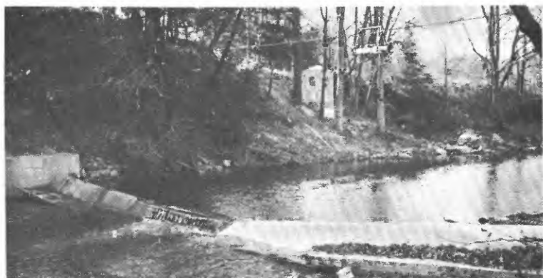
C, MILL RIVER AT NORTHAMPTON, MASS.
