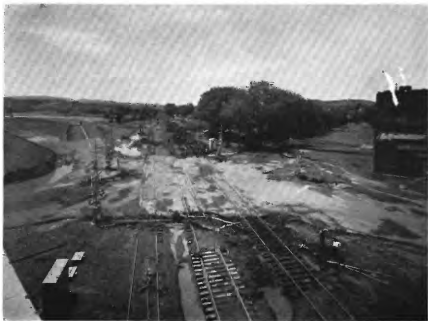
B. Mud and debris on A.T. & S.F. Ry. tracks upstream from U.S. Highways 85 and 87 overpass. Photograph by Corps of Engineers.
