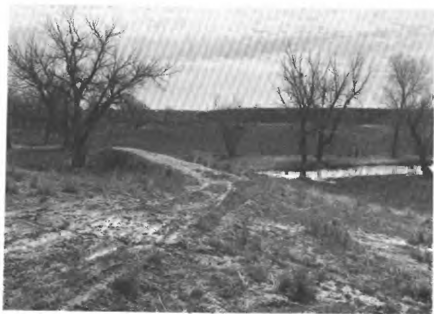
FIGURE 2.—Two views of the valley of Box Creek showing typical dikes used to divert flow from channel and irrigate the flood plain.
