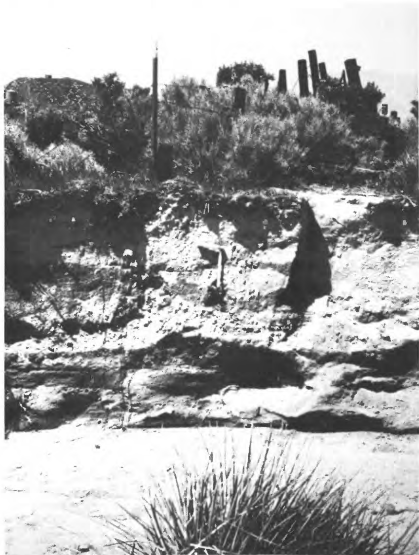
FIGURE 15.--Downcutting of a tributary to Cañada de los Alamos near Kinsey Ranch. Channel was a shallow swale prior to March 1978. The channel was about 5 ft deep and 30 ft wide in April 1978.
