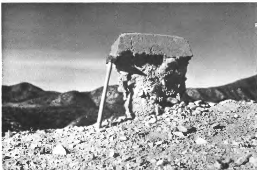
FIGURE 11.--Severely eroded benchmark on "Bench Mark Hill" in January 1976. This benchmark had been eroded out and, by April 1977, had rolled down the hill. Photograph by Howard Wilshire, Geologic Division, U.S. Geological Survey.
